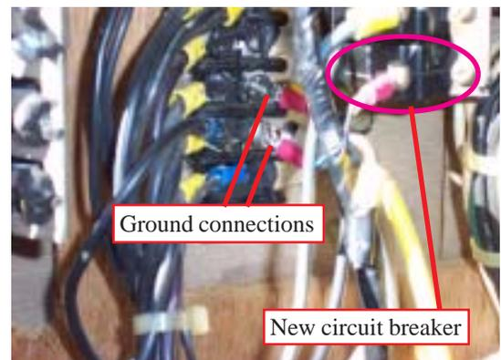
**Fig 11 - Power tee connection to circuit breaker panel**
