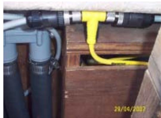
**Fig 12 - Power tee connection to display and transducer**
