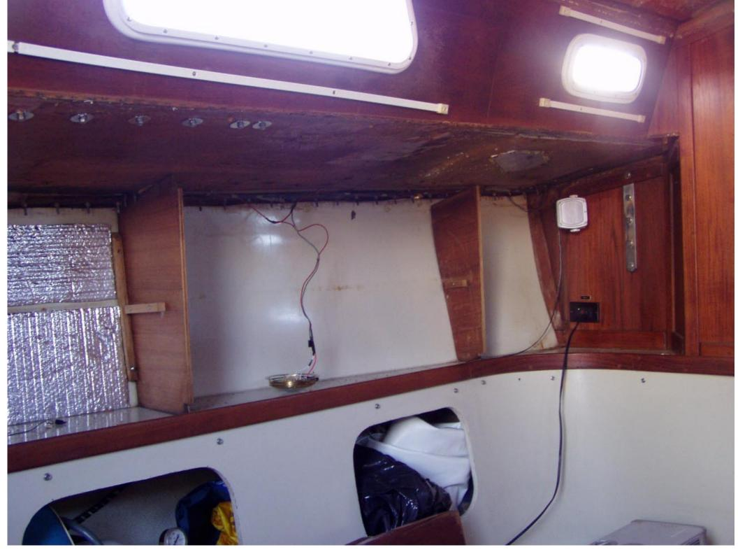
Port side cabinetry remover in order to insulate hull, deck and coach top
